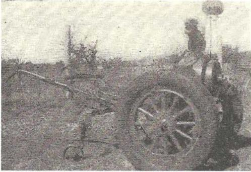
A check is winging its way to Edward Hutson of Muskegon, Mich., for his home built garden tractor. Axle, wheels, frame and handles were made from parts of a Model T Ford. The power is supplied by a Delco light plant air cooled motor. The width of the tractor is 32 inches, and it has a clearance of one foot. A transmission with a 50 to one ratio is used to reduce speed to a slow walk. The motor is connected with the transmission by a belt fitted with a tightening lever that operates as a clutch.
