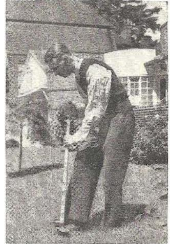
A scientific lawn aerator or sod spiker loosens the sod from underneath and cultivates the soil, thus making the lawn porous without tearing or disturbing the grass.
