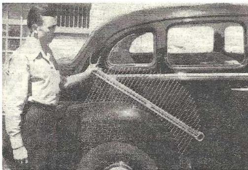
For measuring difficult contours on autos, planes or boats a tool with 34 feelers has been devised. When placed on any curved surface the feelers automatically fall into place and are kept in an accurate outline by locking the handle.
