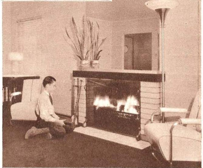
The efficiency of the living room fireplace is multiplied at least four times by a polished aluminum reflector placed behind the grate.
